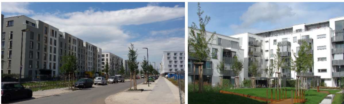
Figure 10: View of some buildings in the Bahnstadt district (Pictures: PHI)
