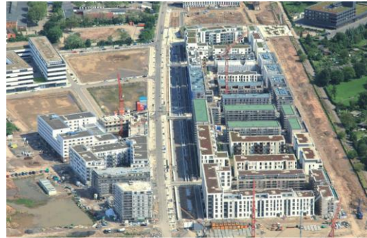
The “Bahnstadt” in Heidelberg (Germany) is the world’s largest Passive House district. At the International Passive House Conference 2014 it received the “Passive House Award” (in the category “regions”) for its exemplary nature. Source: PHI
