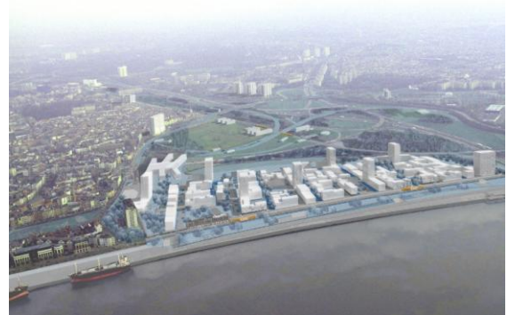
The Nieuw Zuid development in Antwerp, Belgium: an example of urban district designed entirely according to the Passive House Standard within a successful mode of publicprivate partnership. Source: Studio Associato Secchi - Viganò
