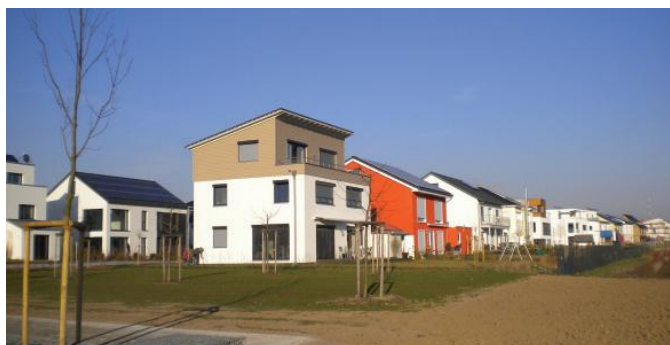
A new Passive House settlement in the PassREg frontrunner Hannover: the zero:e park, the European largest zero-emissions development ( http://www.zero-e-park.de/en/home/ ). Source: Matthias Wohlfahrt, proKlima
