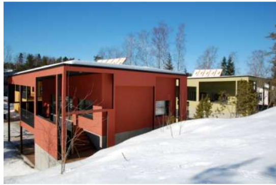
Oravarinne Passive Houses (Espoo, Finland). Foto: Kimmo Lylykangas Architects
