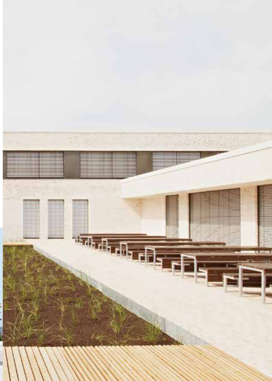
Photos: Riedberg Secondary School | Frankfurt am Main | Architects Ackermann+Raff | Germany © Thomas Herrmann
